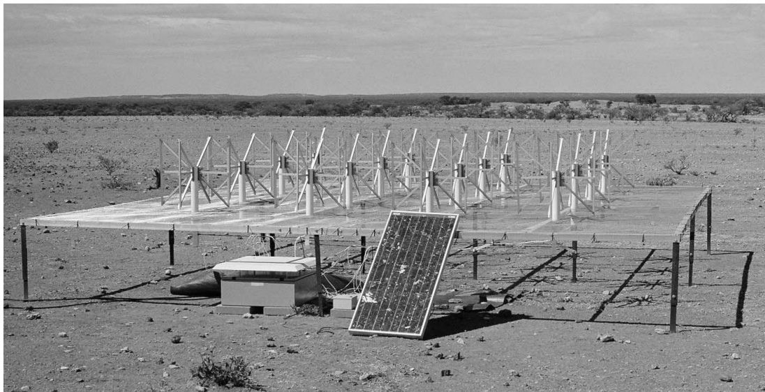
FIG. 1.—Photograph of the first MWA prototype antenna being tested on site in Mileura. The antenna consists of 16 crossed dipoles in a 4 \times 4 m grid, and is elevated approximately 0.5 m above the ground. Five hundred antennas will be placed in a 1500 m diameter array for the low-frequency band of the first-generation MWA. [See the electronic edition of the Journal for a color version of this figure.]
